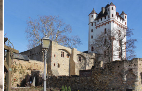
Electors' Castle, South facade
